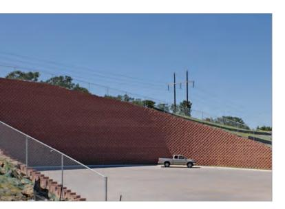
mum NCMA and AASHTO standard is only 1.3," said Miller. "The major difference in building a wall with these more-stringent standards is the use of substantially greater amounts of geogrid. The design called for granular backfill to be hauled in from offsite. And a drainage system was also required to address groundwater levels threatening the base of the wall."
