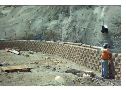
After those nails were placed, the sacrificial nail had to be sealed. Each boring was pressure grouted until all of the air was removed. This process ensured that the galvanized nail did not erode due to moisture contact. The slope face was then shotcreted to prevent erosion or slope failure. Next, the top half of the ramp was removed in order to access the middle portion of the slope and the soil nailing and shotcreting process was repeated.
