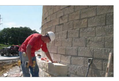
In order to flex, expand and contract as a cohesive system, the limestone veneer was dry stacked in front of the Keystone wall to which it was attached. The limestone veneer was attached to the Keystone Compac Straightface units with a Tapcon™ screw and a stainless steel, "z-shaped" strap system.
