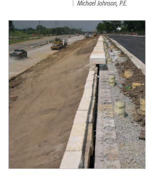
approximate dimensions of the limestone blocks were 12 inches high, by 30 to 36 inches wide, by 14 inches deep. The Keystone Compac wall was assembled in a near-vertical configuration to a maximum height of approximately 10 feet along the 465-foot length of the structure. Behind the Keystone wall, a four-inch perforated PVC drain-tile with sock was installed to assist with water flow through the crushed stone fill.
